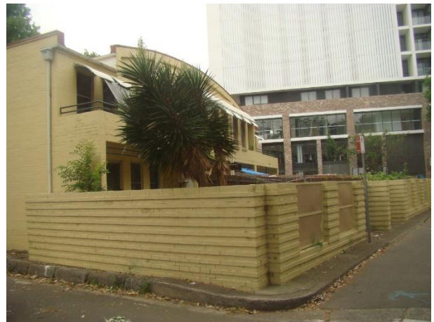
Figure 24. Rear of 2A-2D Wentworth Park Road.
